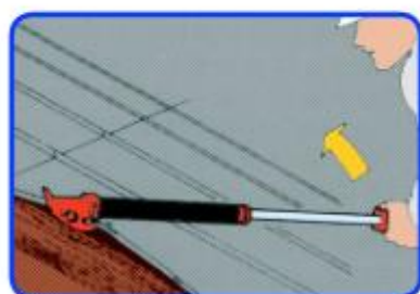
7. Breaking up roof, sheet metal.
